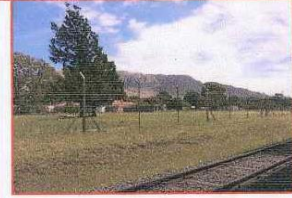
The railway line connecting the silos to the grain store.
