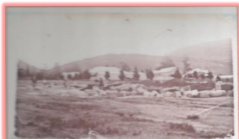
Front of the Postcard where the Foundation is being laid. The Builder is at the left front.
