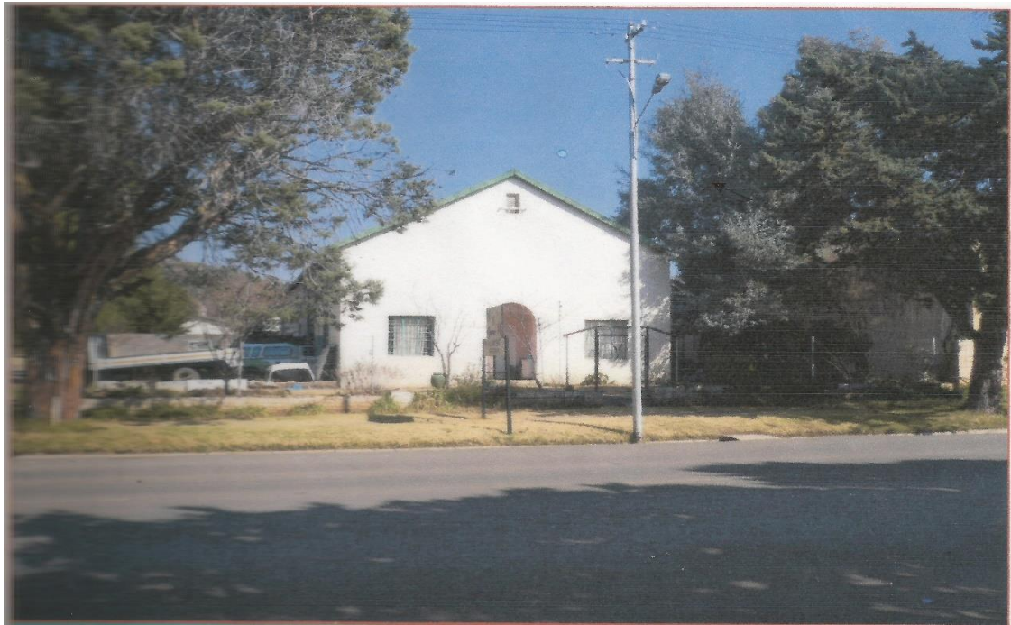
Tant Hessie se "Skating Hall", soos dit al die jare en vandag nog lyk Tant Hessie's "Skating Hall" as it appeared through all the years, till today
